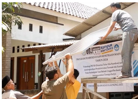
Gambar 5. Pemasangan solar panel 660 WP
