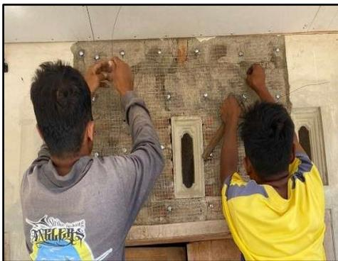
**Gambar 12.** Pemasangan Wiremesh
