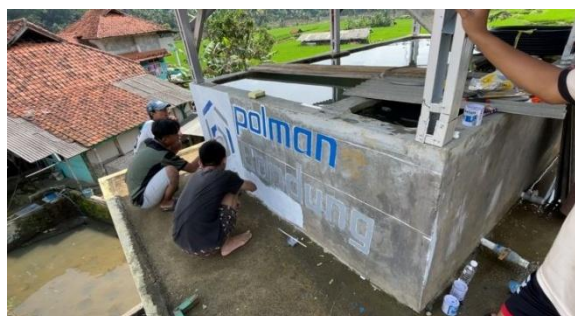
Gambar 6. Proses pengecatan bak water treatment
