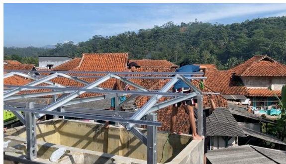
Gambar 5. Instalasi atap bak water treatment
