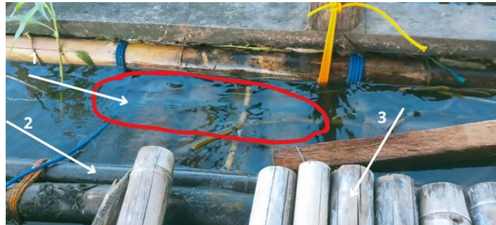
Figure 3. Raft layers of a community Bola Rai' floating house.
